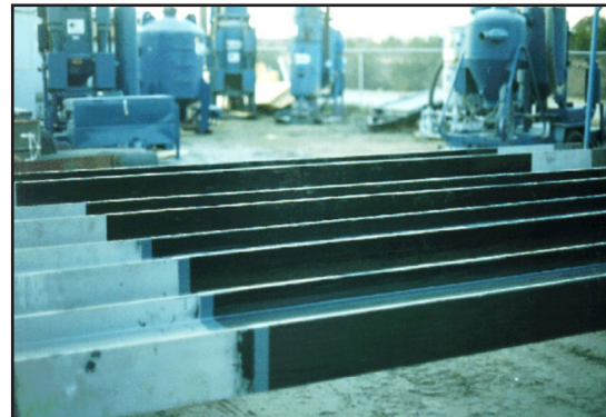
Two coats of ARC 855 - the end to be coated after welding
